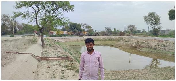
It had much lower water holding capacity than its original potential. This was primarily due to the improper maintenance and lack of connection of supply channel to the water body. Desilting or deepening of these water bodies has never been carried out for the past few years.
